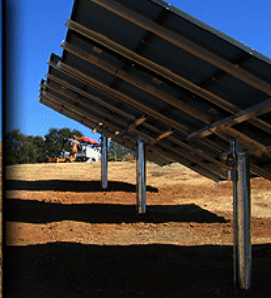
Example 2: Hillside pole mounted fixed PV installation.
