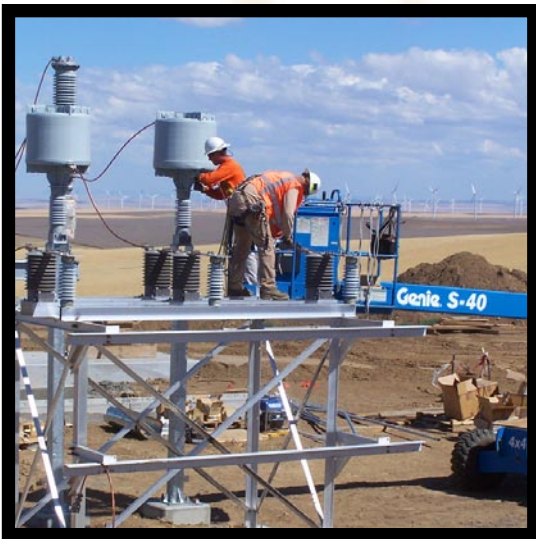
Electricians wiring switches and reactors at wind farm substation. Photo credit: John Demoss
