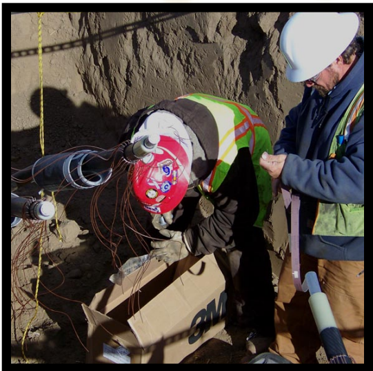
Technicians prepping wind turbine transmission cables for splice. Photo credit: John Demoss
