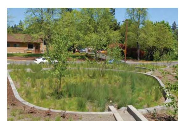
**detention** temporarily holding back stormwater before releasing into the sewer system
