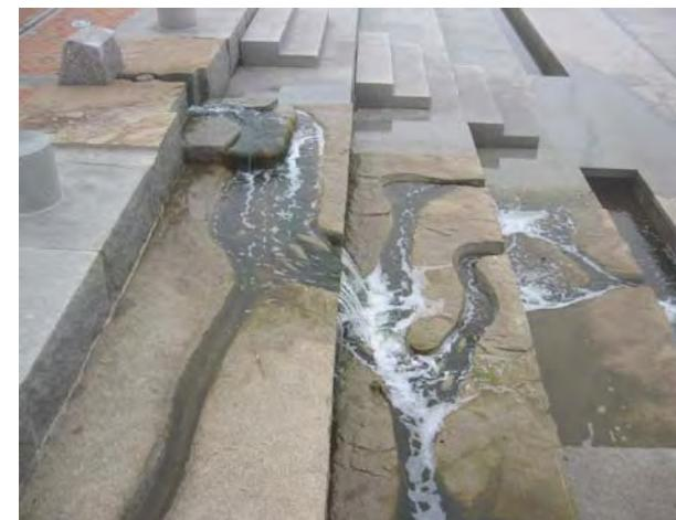
**conveyence** the transport of stormwater from one point to another
