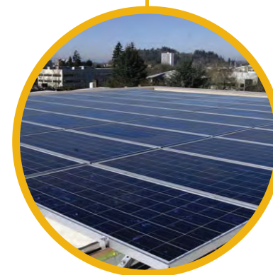
monocrystalline panels for renewable energy and solar hot water
